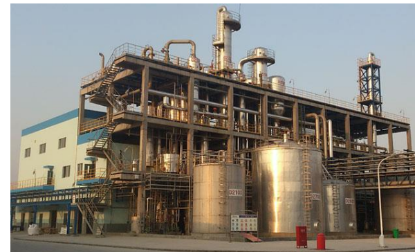
The new Neo plant in operation
